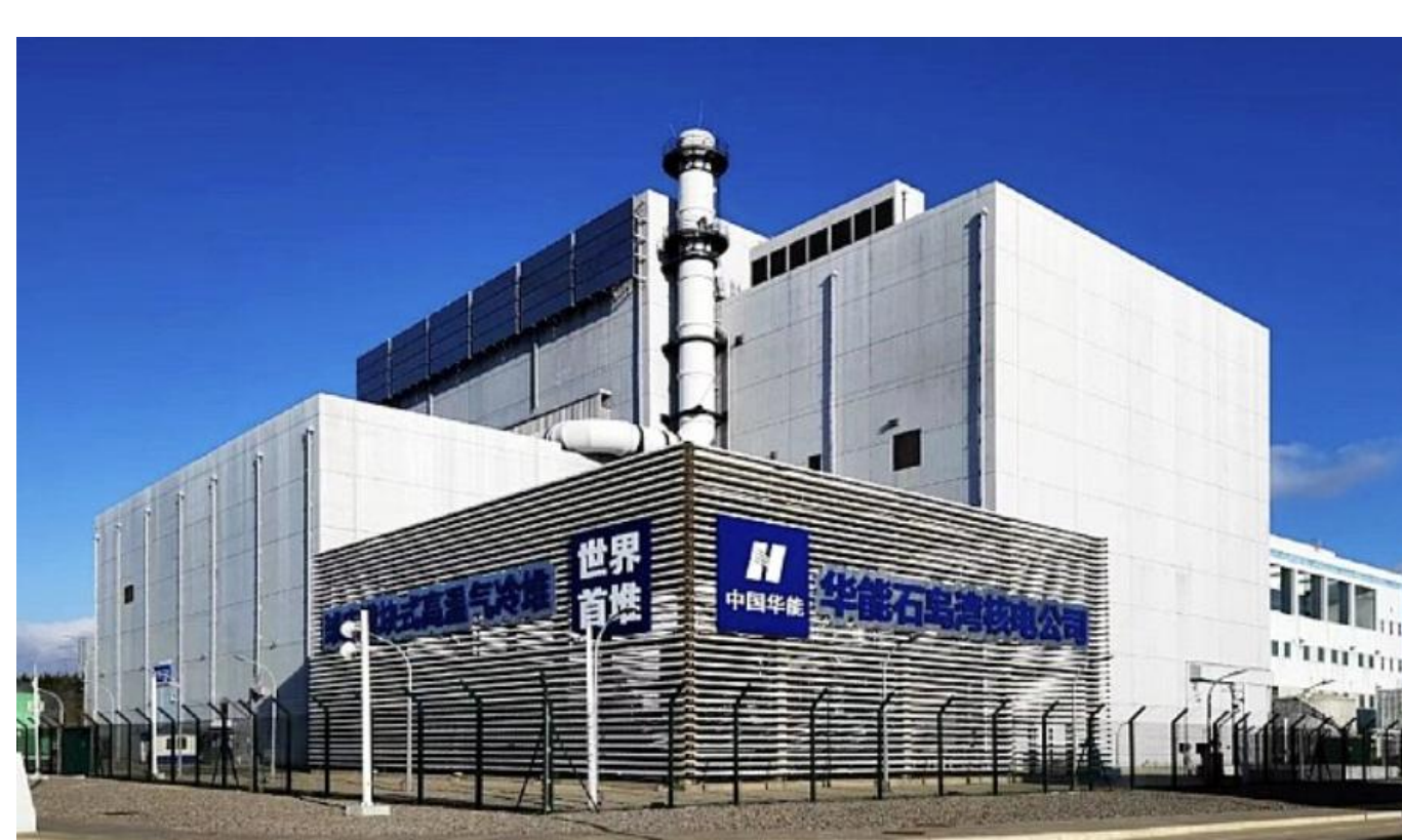
Two 250 MWth HTR-PM modules coupled to the grid since December 2023
